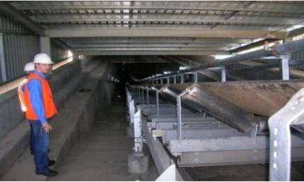
➤ Each conveyor is driven by 2 motors in master-slave connection. One 900 kW motor in the head and one in the tail; the communication between inverters and PLC is controlled via Ethernet.
