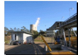
Centrale termoelettrica Thermal power station
